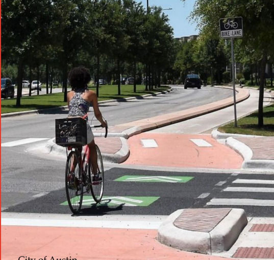
Vertically separated bike lane using a concrete curb in Austin, TX, USA that considers context in selection of facility type. Source: City of Au.
